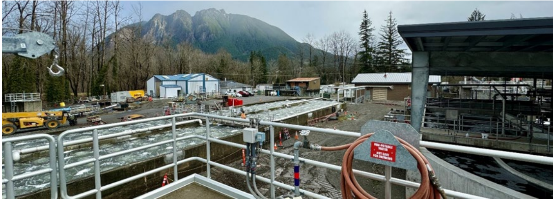
Figure 1 Wastewater Treatment Plant (2024)
