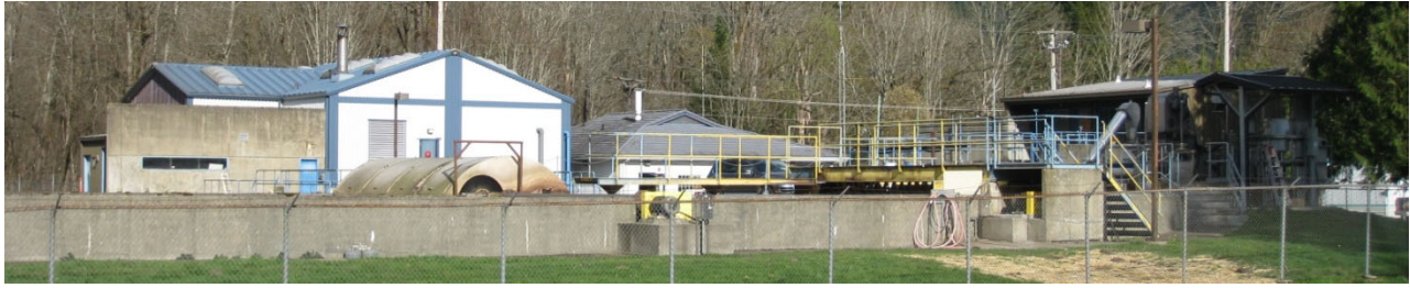
Figure 1 Waste Water Treatment Plant (add photo credit with date update photo)
