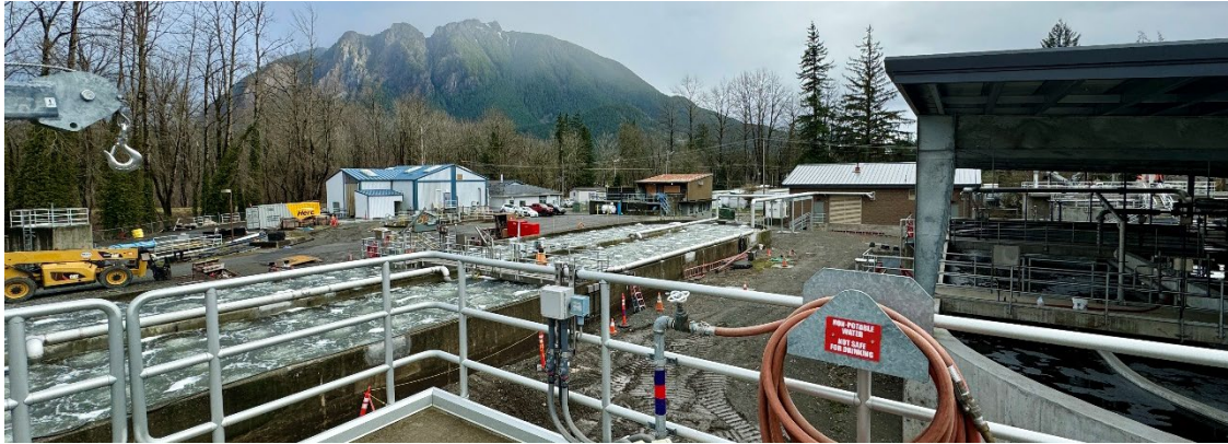
Figure 1 Wastewater Treatment Plant (2024)
